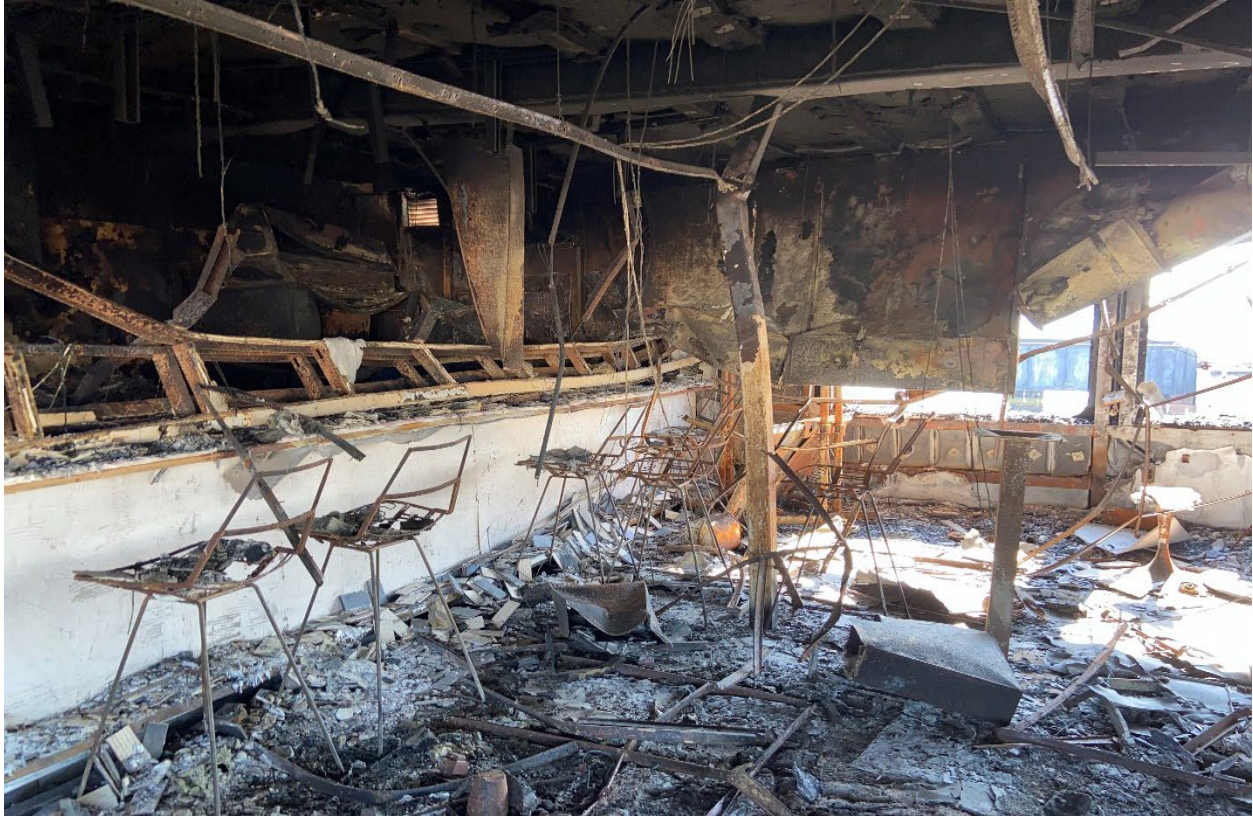
Harborview Deck. Source: USCG.
