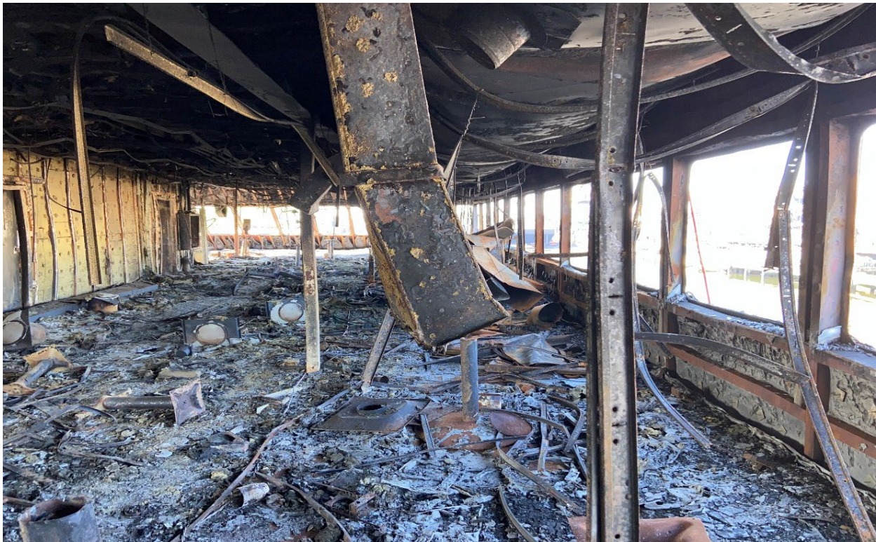
Harborview Deck. Source: USCG.
