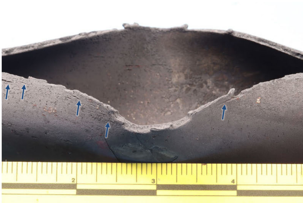
Figure 7. Oblique view of the pipe B fracture showing step features in the fracture plane corresponding to longitudinal crack-like pits (indicated with unlabeled arrows) on the exterior surface.
