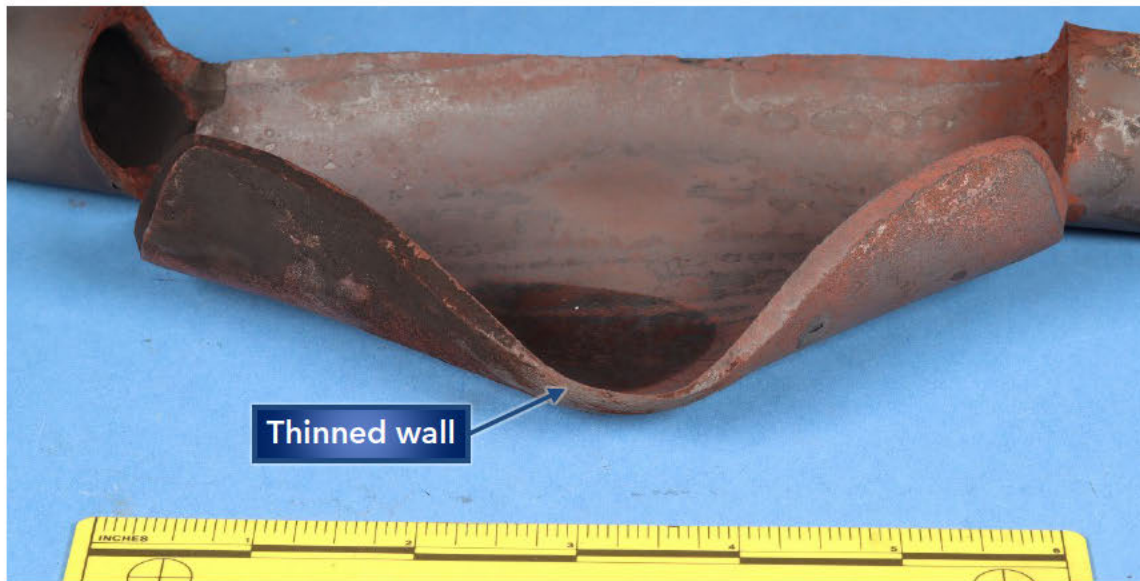
Figure 4. View from the lower side of pipe A showing wall thinning at the center of the bulge in the fracture location.
