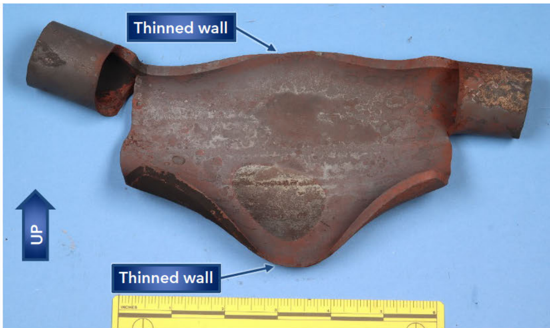
Figure 3. Closer view of the pipe A fracture after sectioning and partial oxide removal. Areas of reduced wall thickness at the fracture location are indicated.
