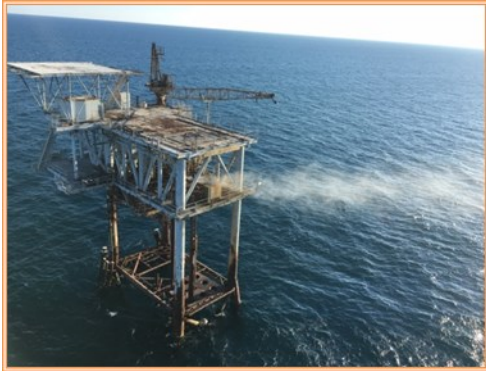
Above: Abandoned MU818 Natural Gas Platform 3.5 miles offshore spraying natural gas and condensate.
