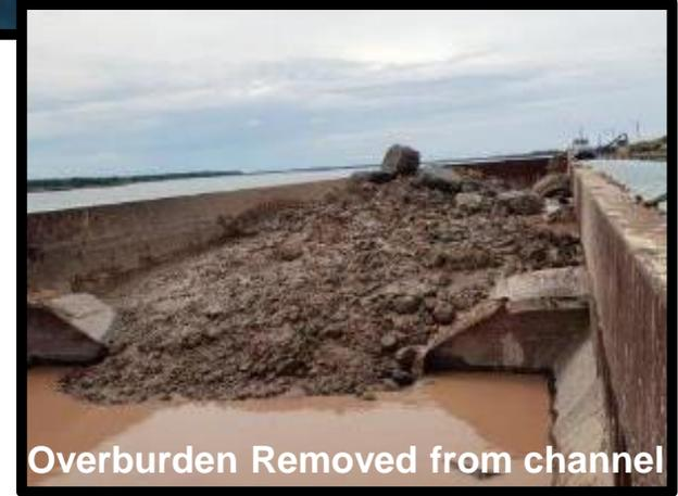
**Scope:** Remove 250,000 CY of Jacobsville sandstone and overburden to deepen the Upstream Approach Channel to depth of 30 feet
