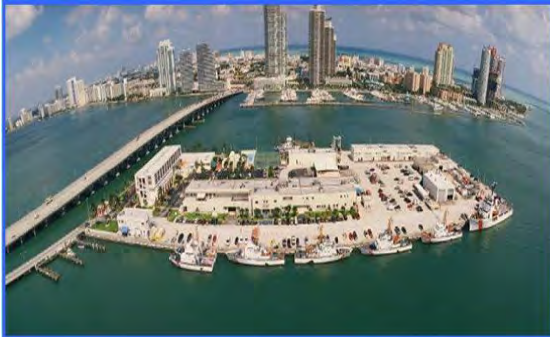
Figure 2 - USCG Base Miami Beach looking east
