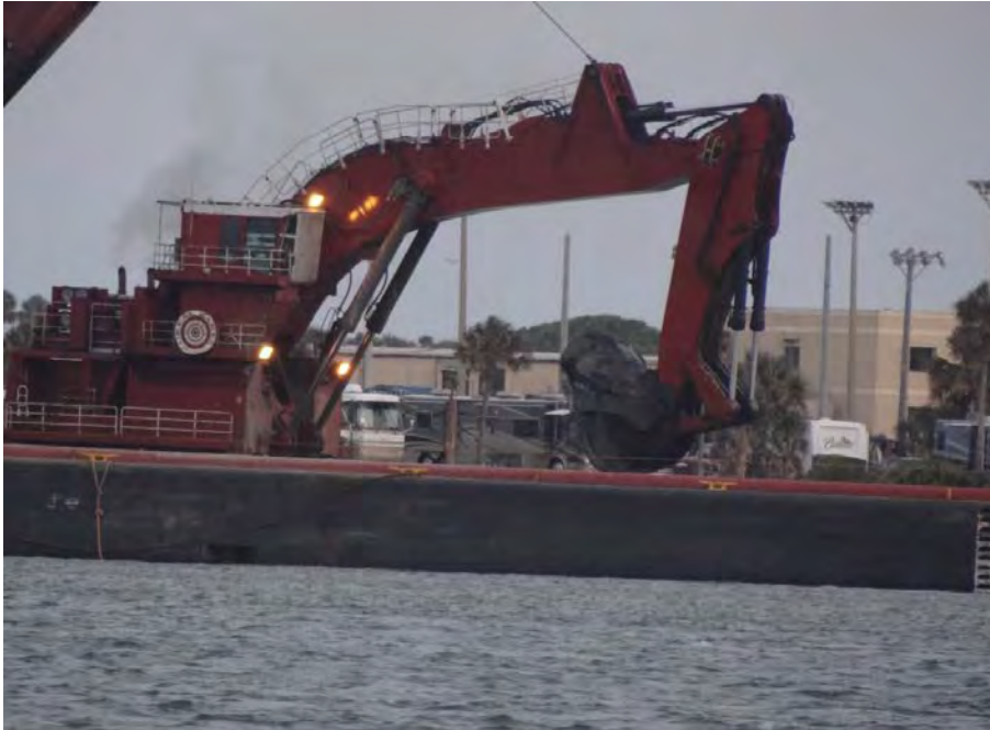
Figure 11 - Backhoe loading a scow
