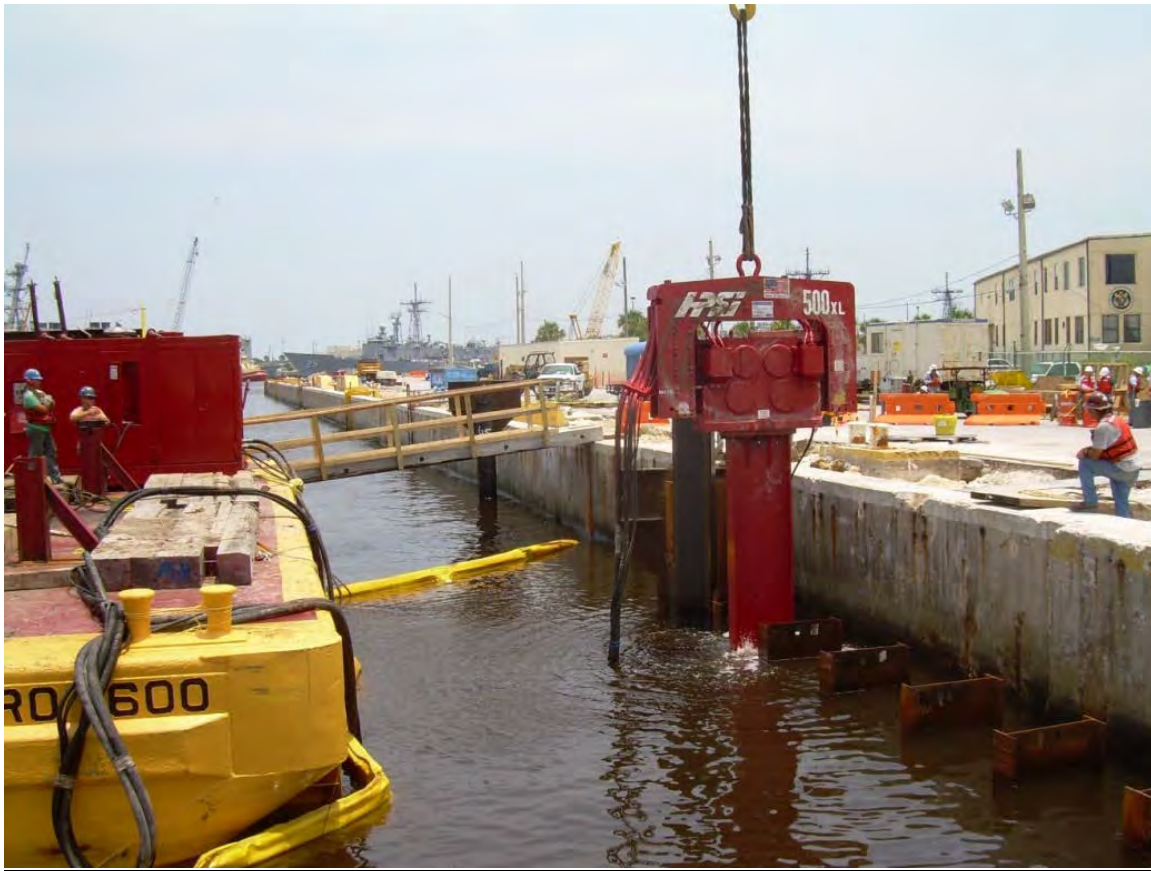
Figure 5. Vibratory Installation of Sheet Piles at NAVSTA Mayport
