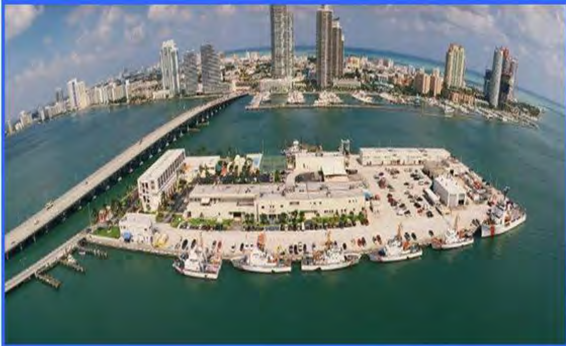
Figure 2 - USCG Base Miami Beach looking east
