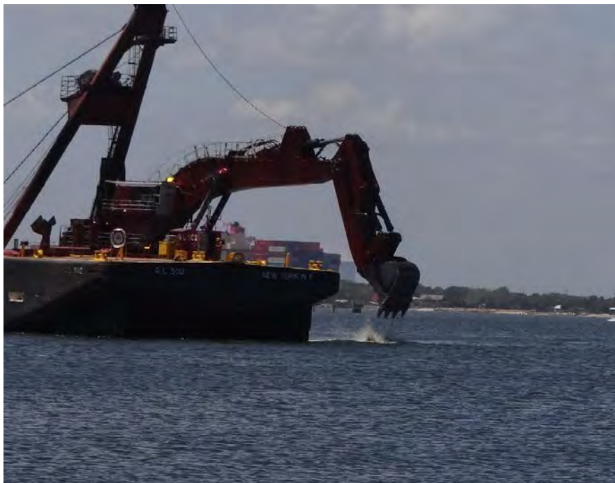
Figure 10 - Backhoe excavator dredge
