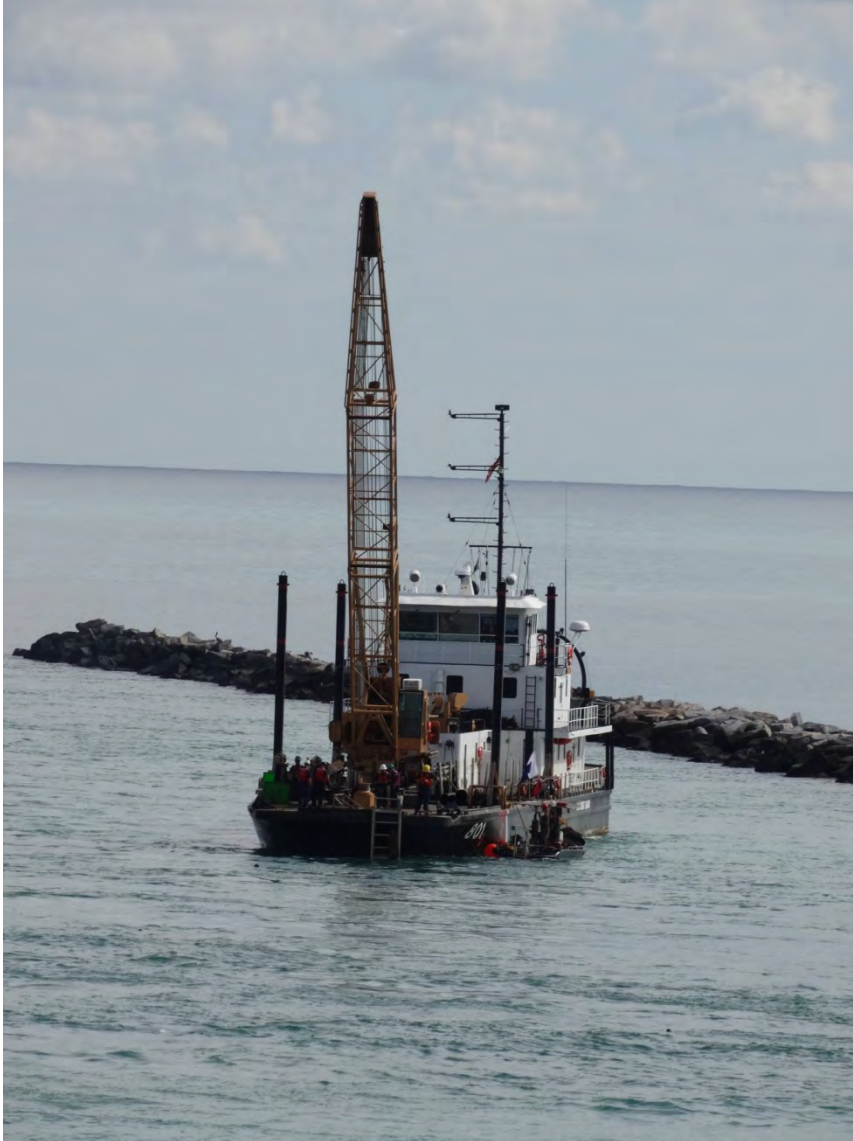
Figure 4 - US Coast Guard Cutter HUDSON repairing an ATON at Miami Harbor
