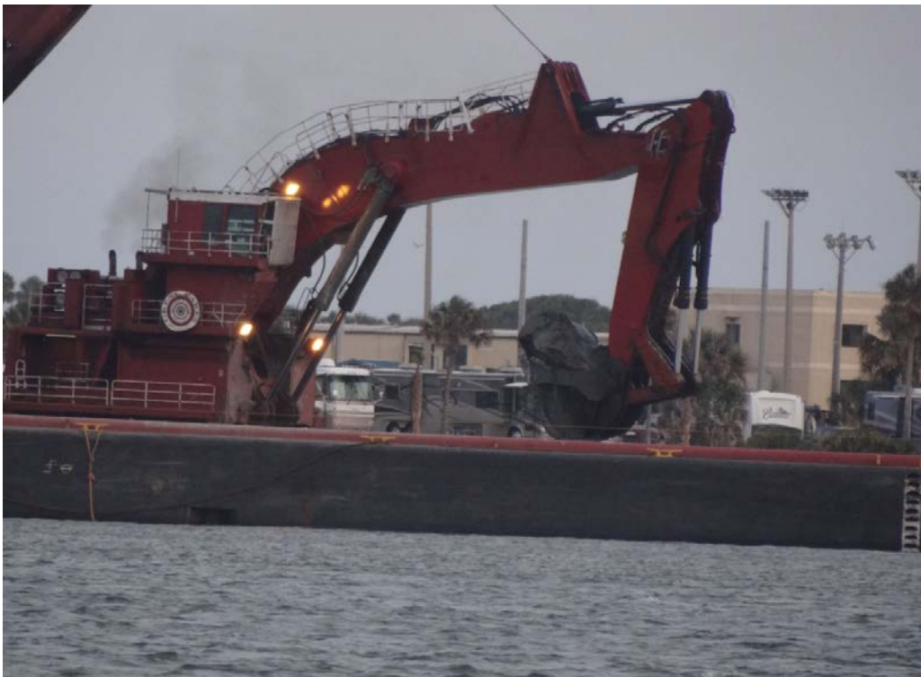
Figure 11 - Backhoe loading a scow
