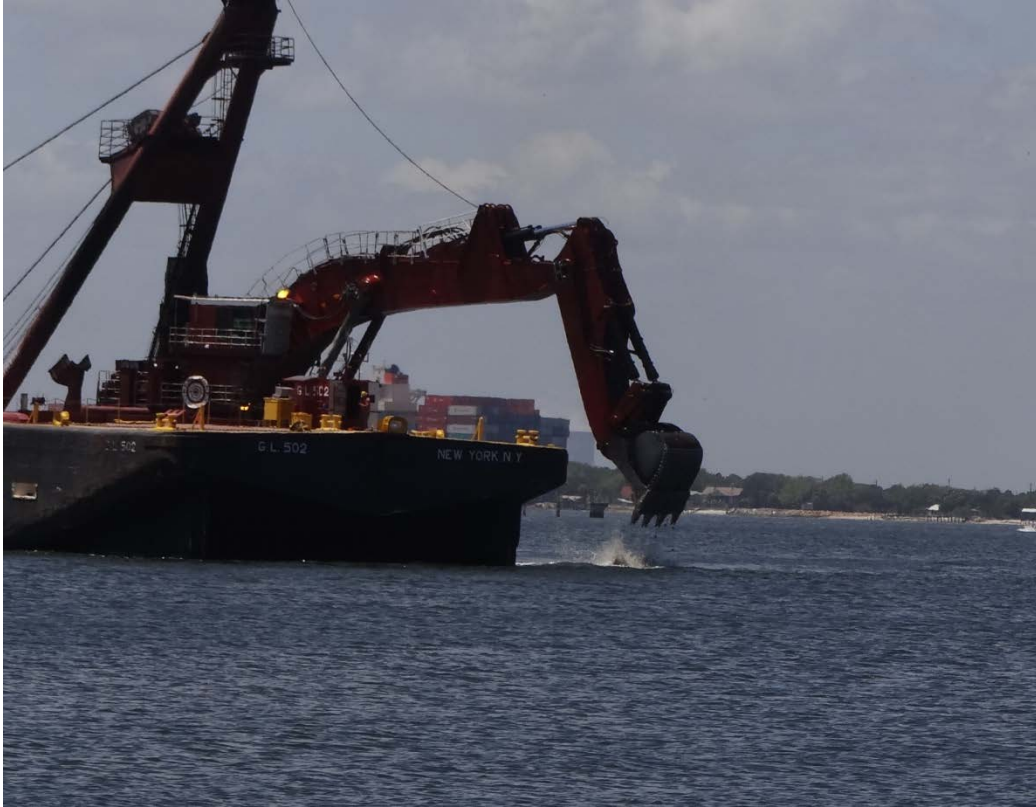
Figure 10 - Backhoe excavator dredge
