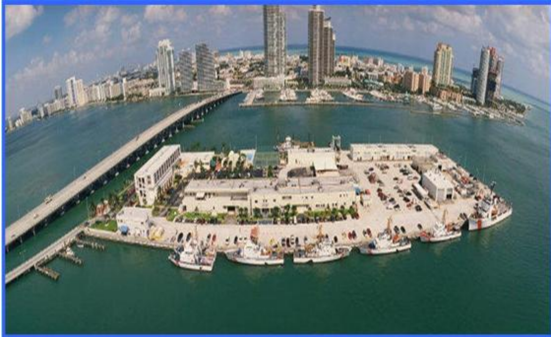
Figure 2 - USCG Base Miami Beach looking east
