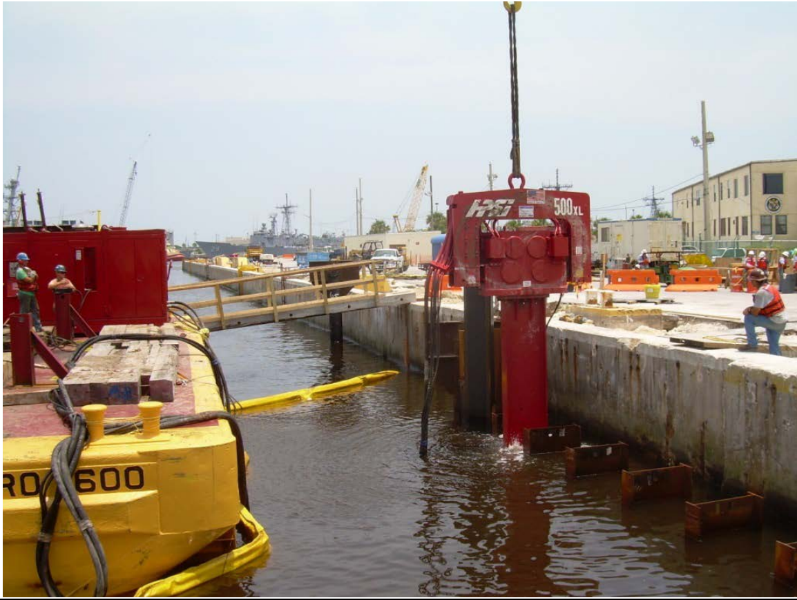
Figure 18 - Vibratory Installation of Sheet Piles
